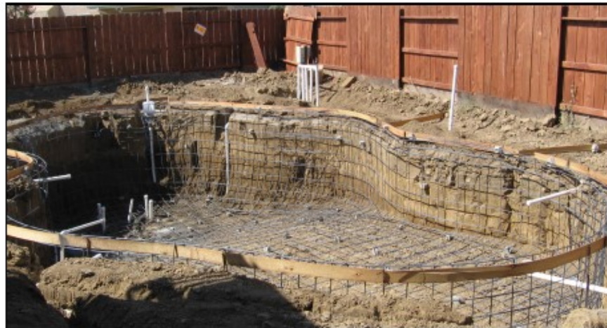
IN-GROUND POOL PRE-GUNITE INSPECTION
