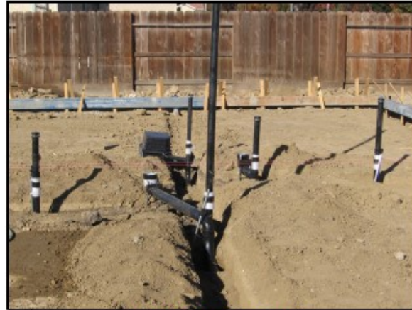
UNDER-SLAB PLUMBING
