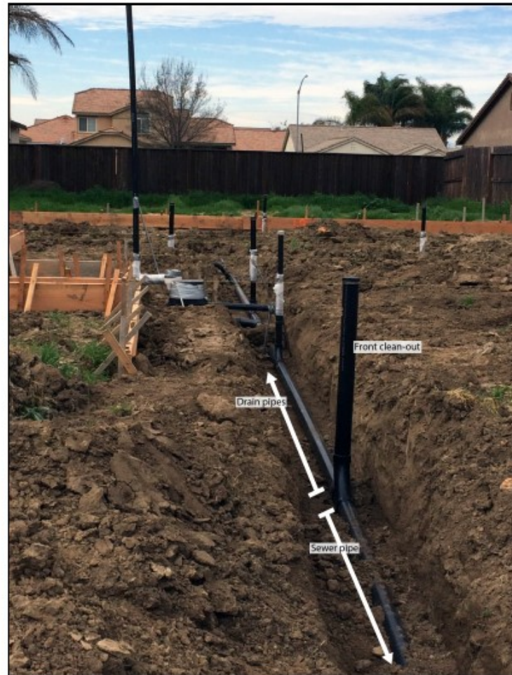
IDENTIFYING DRAIN PIPES FROM SEWER PIPE
