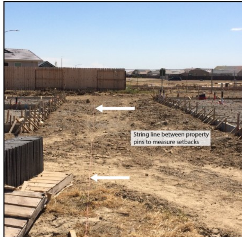
STRING LINE BETWEEN PROPERTY PINS TO MEASURE SETBACKS
