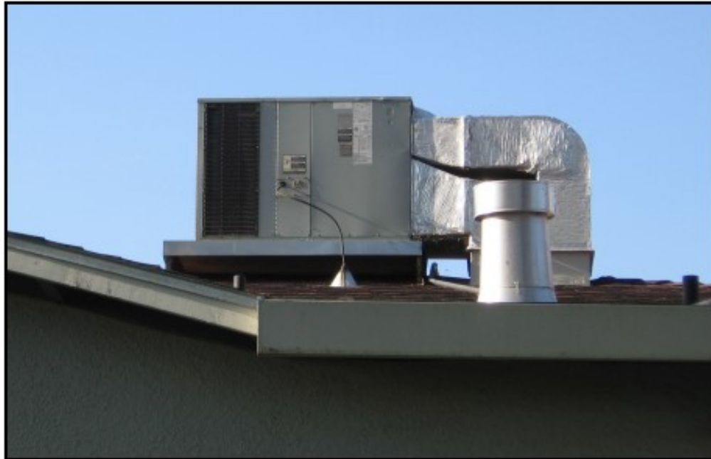
HVAC PACKAGE UNIT ON ROOF
