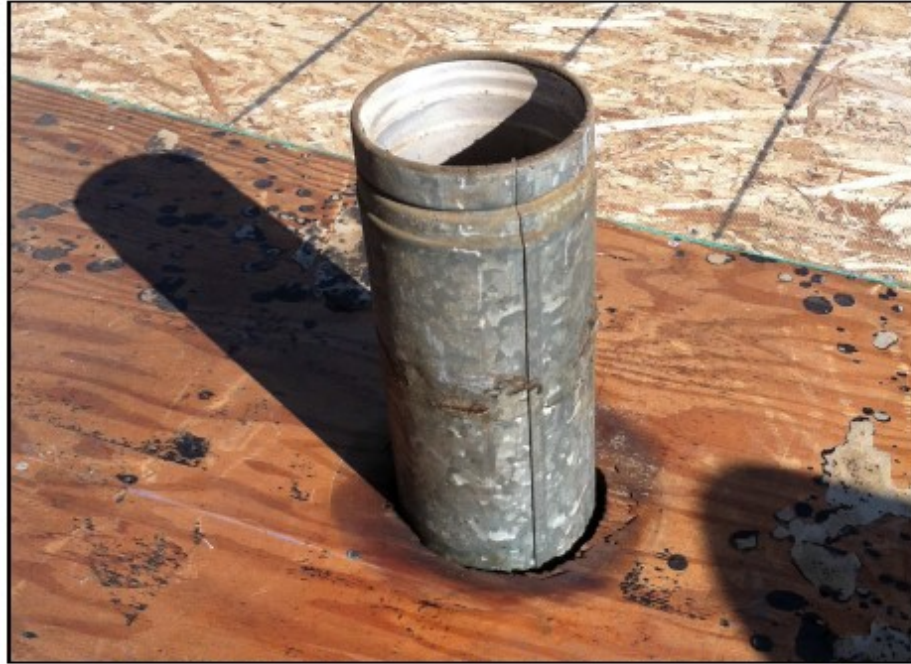
THE REASON WHY CLEARANCE IS REQUIRED AROUND COMBUSTIBLES
