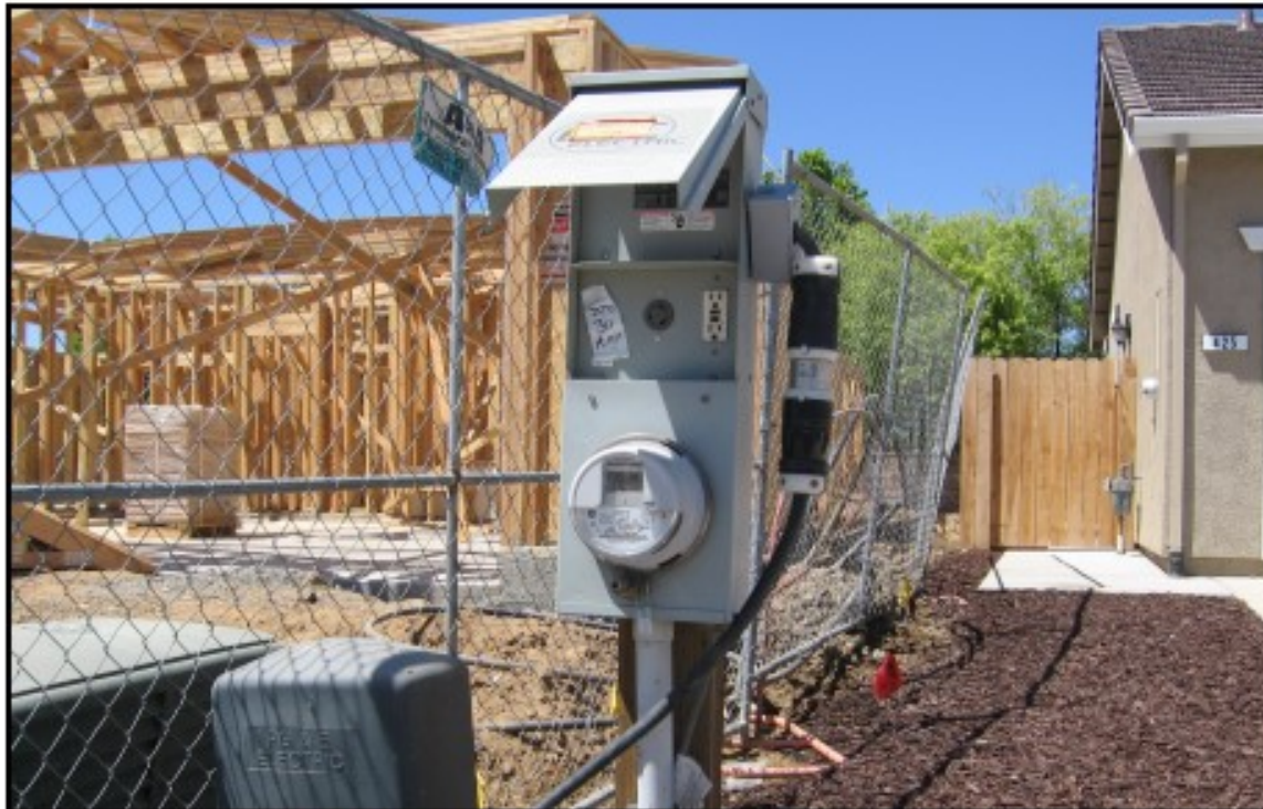
TEMPORARY POWER POLE FOR CONSTRUCTION
