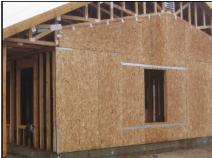
HOUSE READY FOR A SHEAR INSPECTION
