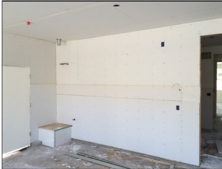
GYPSUM NAILING IN GARAGE
