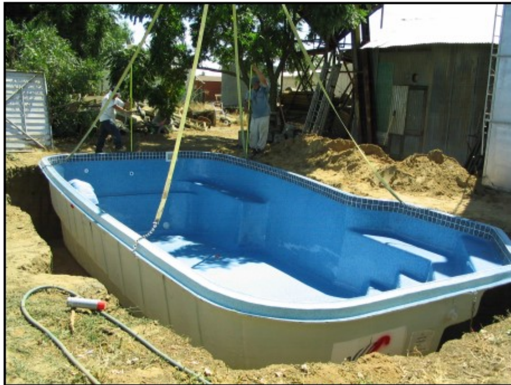
FIBERGLASS/ONE-PIECE POOL SHELL
