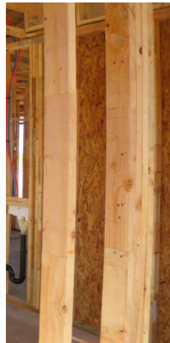
Abutting studs = Built-up column
