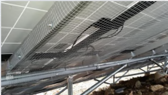
Ground-mount solar array – are wires “guarded”?
