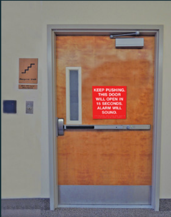
Current delayed egress signage
