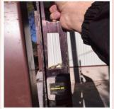
Figure 3.2-1: Non-Acceptable Vertical Tolerance
