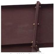
Figure 3.5-3: Snug Tightened Joint
