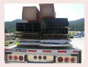
Contractor / Developer / Erector Unloads Metal Building at Jobsite and Stages Materials for Building Erection
