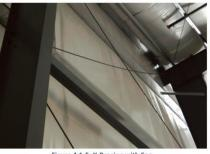
Figure 4.1-5: X-Bracing with Sag
