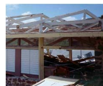
School with Substantial Structural Damage to the Gravity System
