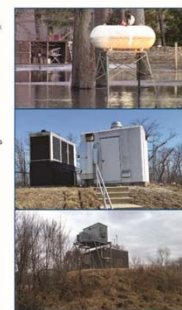
Figure 1: Photos of fuel tanks for a residential area above the flood water near Cedar Falls, Iowa (top); Emergency generator and Emergency Power system for a collector well in Cedar Rapids, Iowa (bottom).
