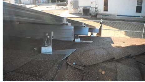
Improperly Installed Flashing
