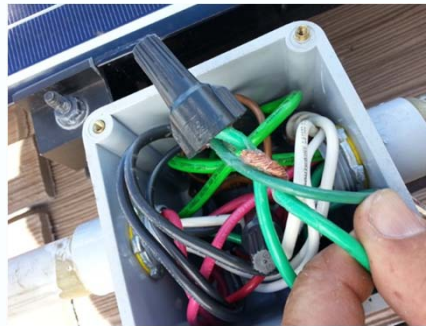
Incorrect Splice of Ground
