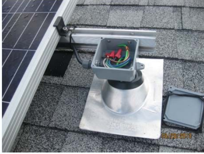
Improperly Installed Flashing
