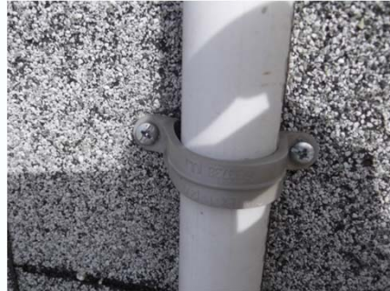
Potential Water Entry
