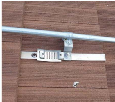
Tile roof conduit support
