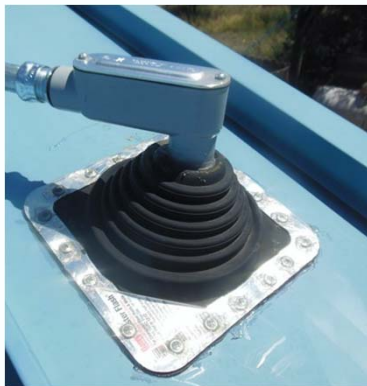
Metal Roof Conduit Flashing and Supporting Options
