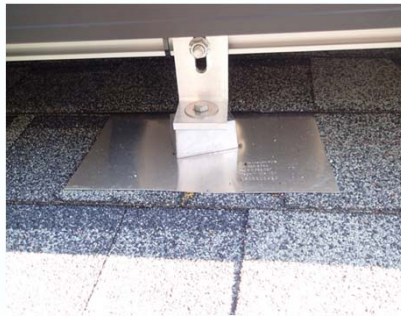
Flashed and Secured
