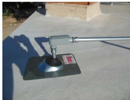
Incorrect Flashing Type
