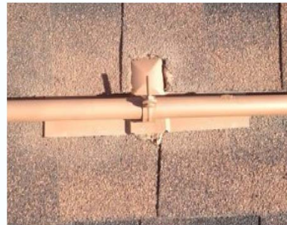
Flashed and Secured
