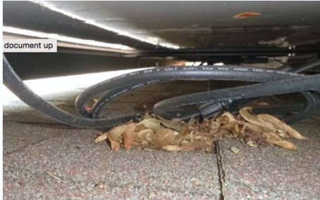
Wires Touching Roof Surface
