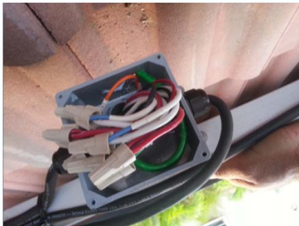
Splice not consistent with conductor rating
