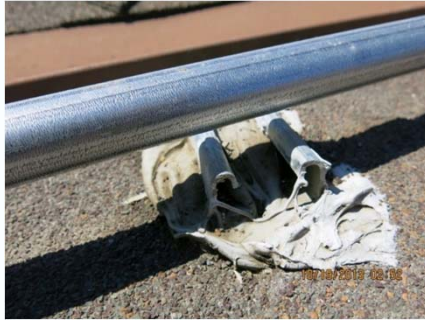
Not Secured; Flashed?
