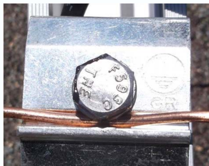
Ground lug on rail
