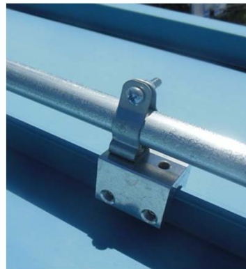
Metal Roof Conduit Flashing and Supporting Options
