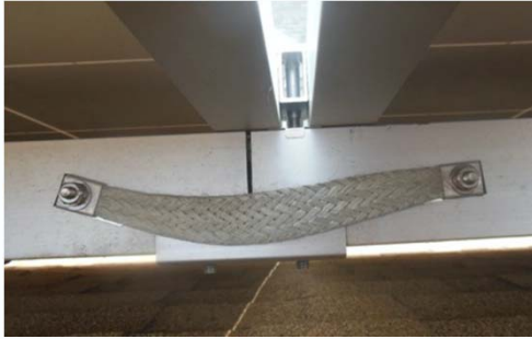
Bonding strip at rails splice
