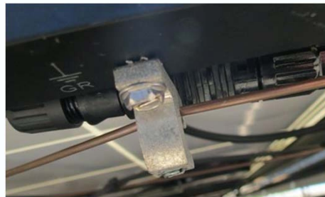
Lug on module with star washer
