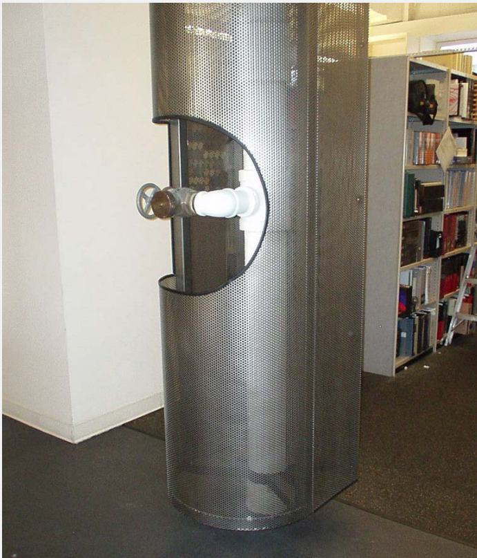
Example of a cowl. Concern with access for fire department and operation.
