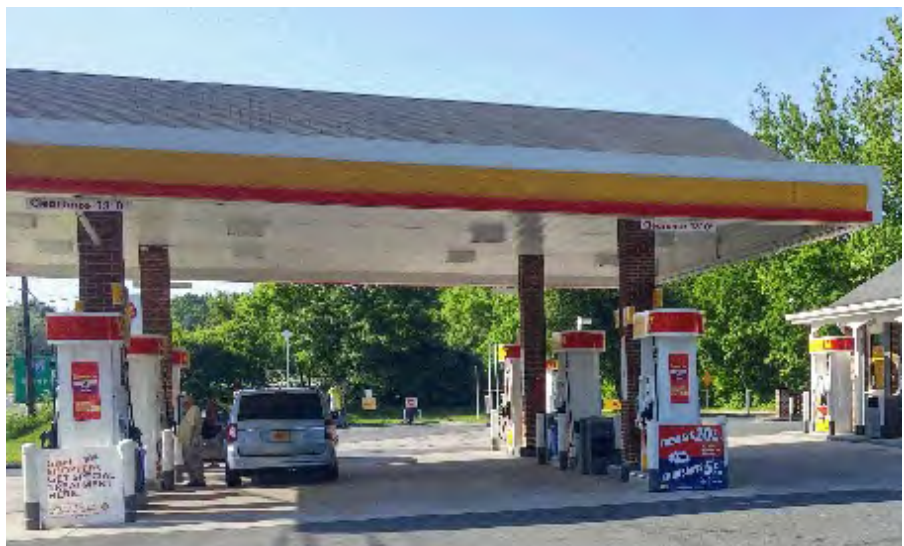
Fuel dispensing island with additional impact provided adjacent to middle dispensers.
