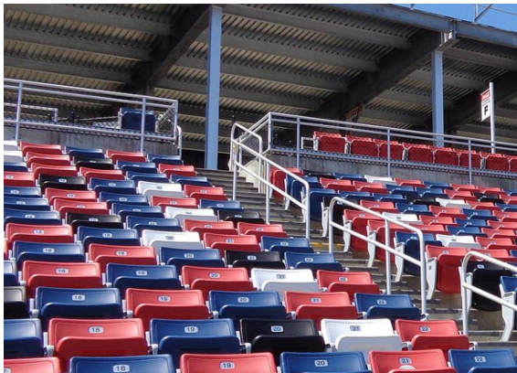
Figure 8 NASCAR Grandstand with mid-aisle handrail transitioning to handrails on each side where there are seats on neither side.
