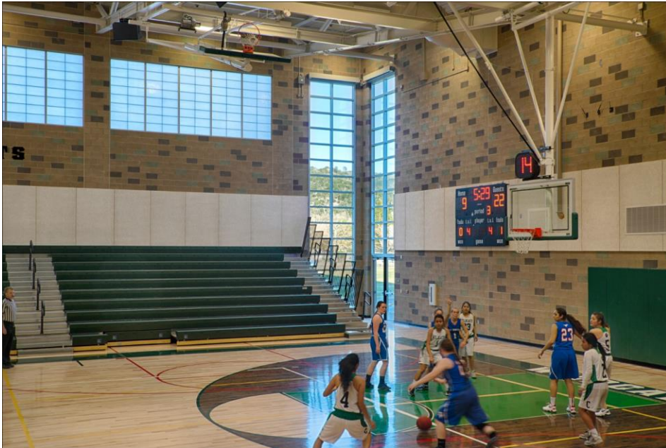
Figure 7 guard does not have graspable handrail at top, so allow for handrail at guard/wall.
