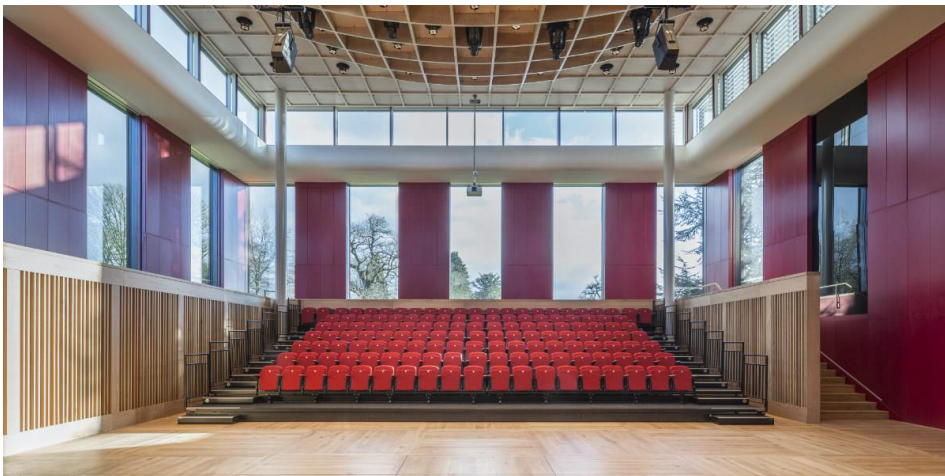
Figure 5 – guard with graspable top rails
