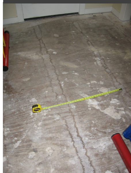
Figure 2. Subfloor with moisture damage in a house with impermeable vinyl flooring (removed) above a vented crawl space
